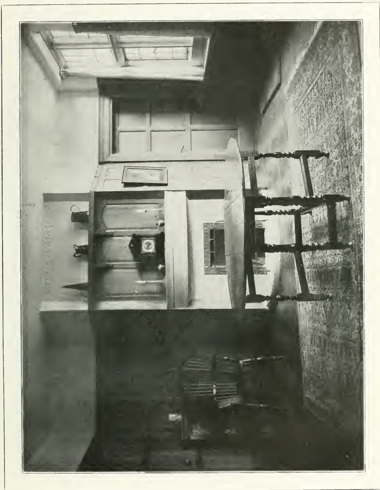
The walls of this room are panelled in oak to a height of seven feet, and the floor is covered with oak parquet. A narrow frieze of modelled plaster takes the place of the ordinary cornice. The chimneypiece is of stone.
